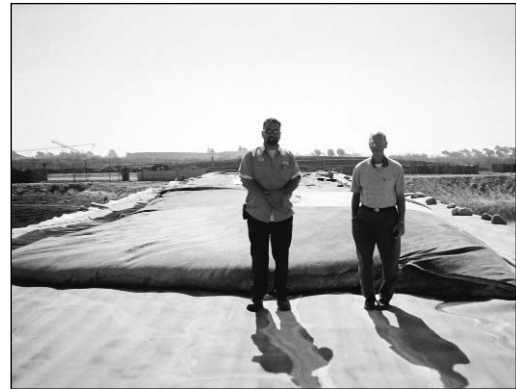
Raudel Juarez, VRSD Operator, and Kelly Polk, VRSD District Manager, stand in front of a Dewatered Geotube® that was filled to a height of 5 feet and allowed to dewater. Solids inside the Geotube® feel like hard clay when walking on the dewatered Geotube®.
