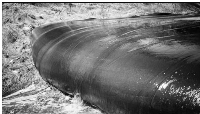
Clean filtrate flows from Geotube® while filling.
