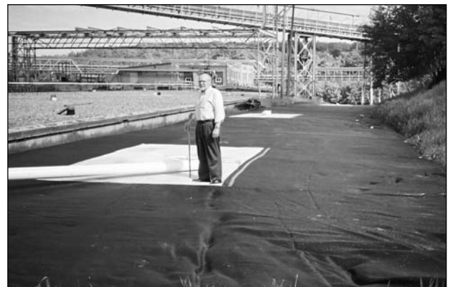
Operations Coordinator, Jeff McCulloch, inspects the dewatering degree of the Geotube® container.
