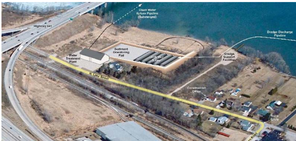
The layout of a dredging operation at Fox River. Geotube® containers are positioned in the center.
