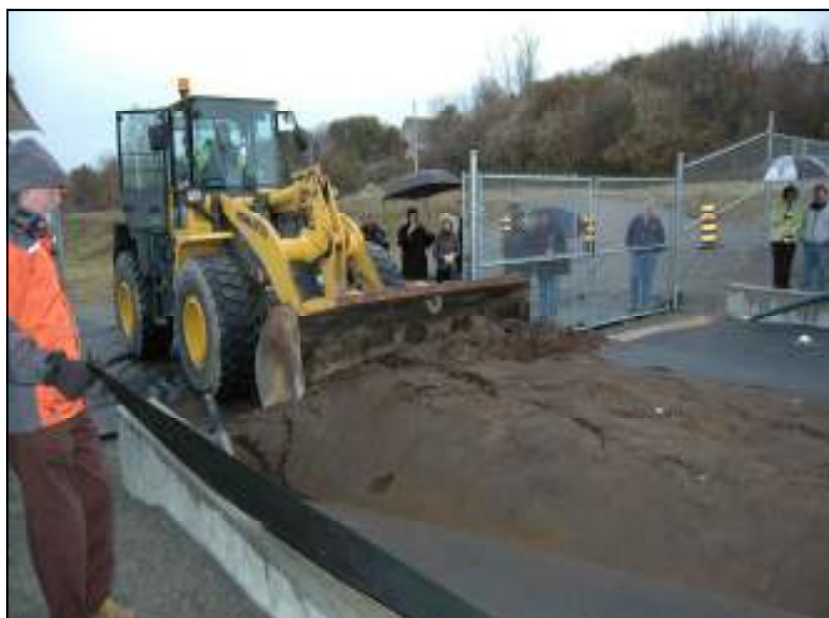
Odorless, dewatered solids are removed from a Geotube® unit in Eganville, Ontario during a Technology Transfer Demonstration hosted by the township on October 27, of 2009.
