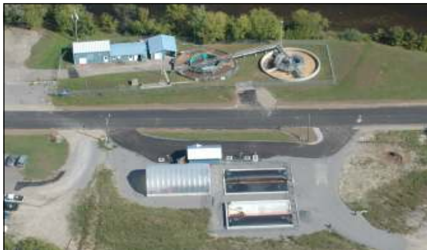
An Aerial view of the Bonnechere Valley Township Biosolids and Septage management which utilizes Geotube dewatering units. The facility has been operational since April of 2007.
